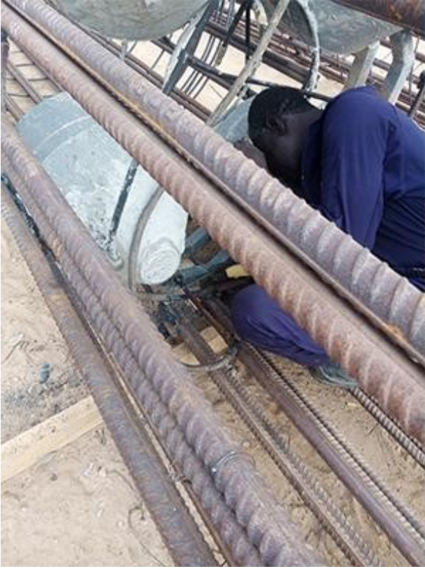
Weld Super-Cell to reinforcing cage
