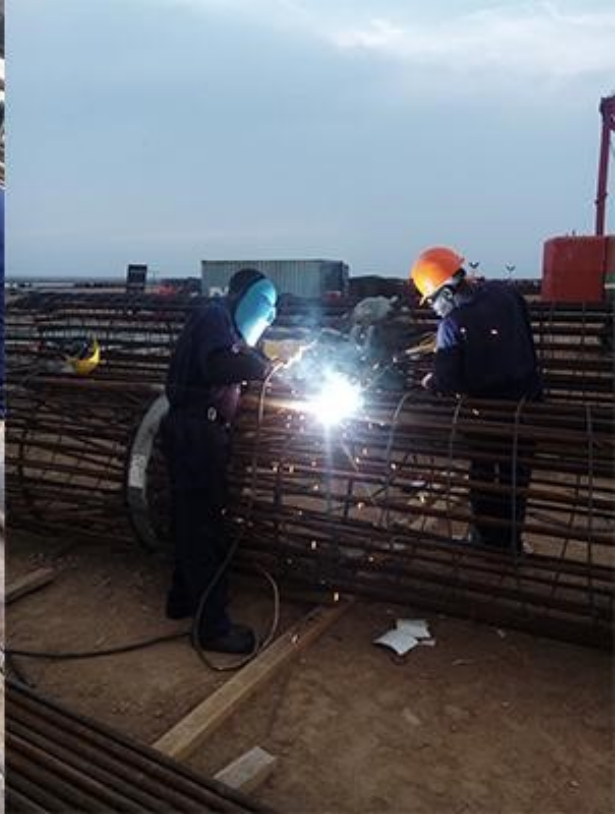
Weld Super-Cell to reinforcing cage
