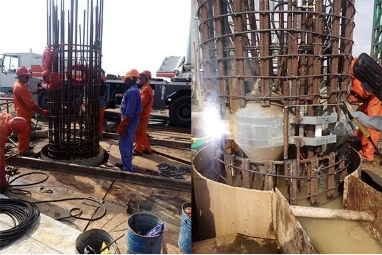
Lifting and installation reinforcing cage 1
