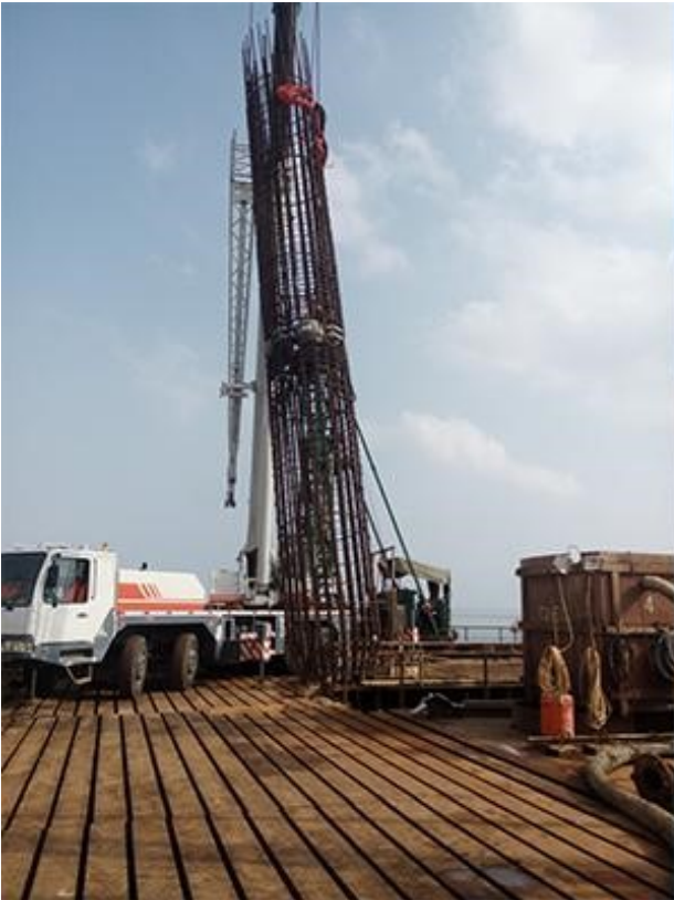
Lifting and installation reinforcing cage 1
