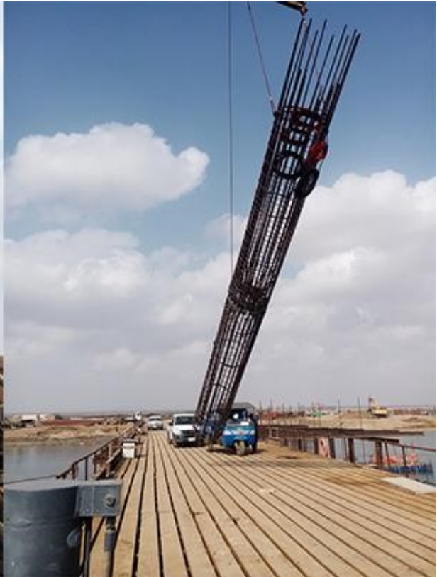
Lifting and installation reinforcing cage 1
