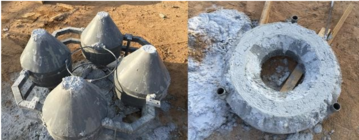
Precast cone-shape flow-guiding mechanism
